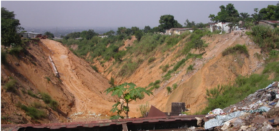
Fig. 2 Mega-gully 'Laloux' has incised Avenue Bolivar over a distance of 2129 km, is about 90 m wide and 30 m deep. The houses, formerly at a certain distance from the street, will slide into the mega-gully as it deepens and widens. In the close foreground, a metallic construction meant to stop headward retreat of the gully head
